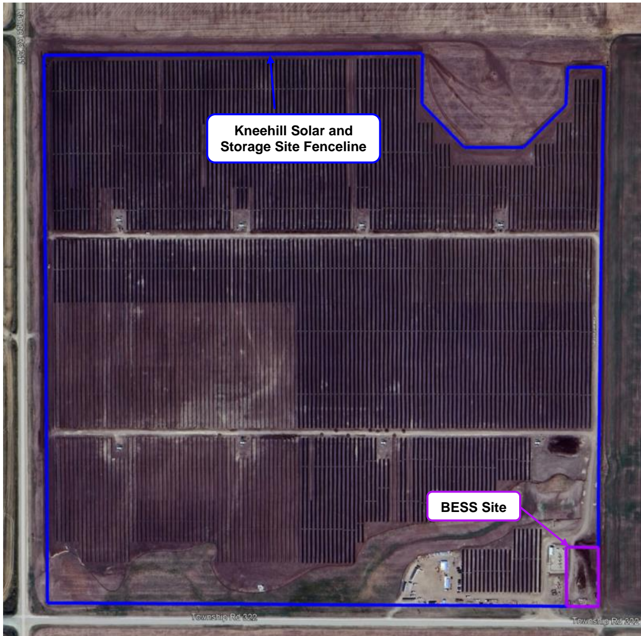
Figure 2 Aerial photograph indicating the Kneehill Solar and Storage Site fenceline and proposed BESS installation site.
